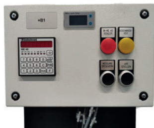
Fig. 3 Control panel with battery level indicator
